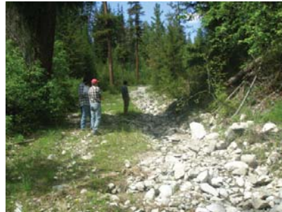
We can see that the road bed has become the stream bed. High temperatures, low dissolved oxygen and siltation are the result.
